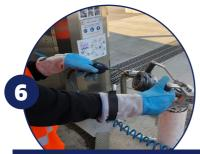
Dry and clean the filler nozzle with compressed air or a cloth.
